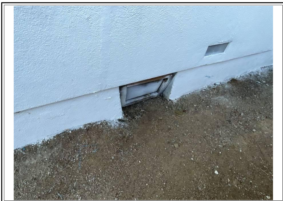
ENTRANCE TO CRAWL
