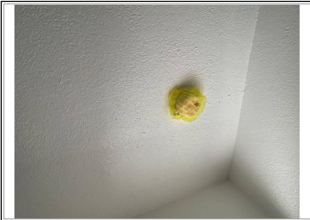
BEDROOM 3 SMOKE DETECTOR
