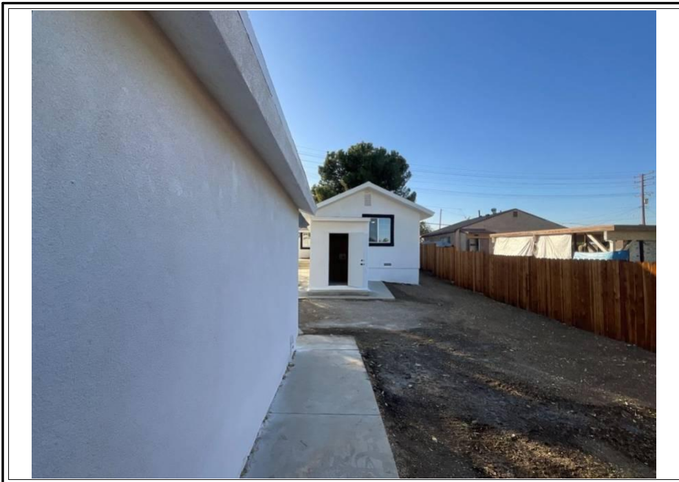
REAR OF SUBJECT PROPERTY
