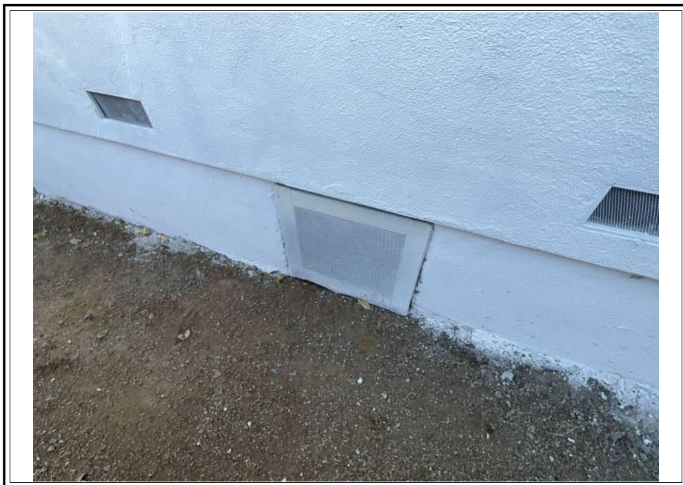
ENTRANCE TO CRAWL
